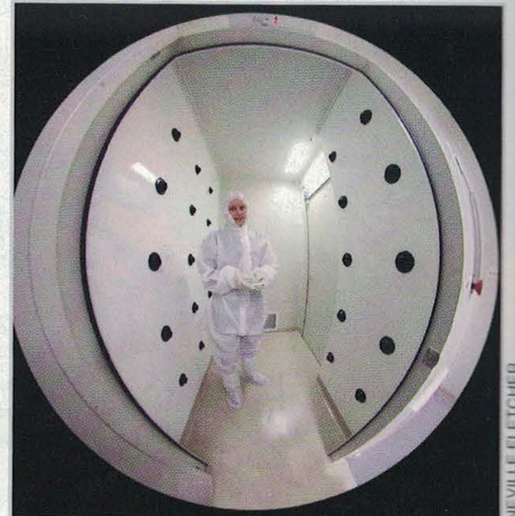
The air-shower entry to a cleanroom at Australian National University.
